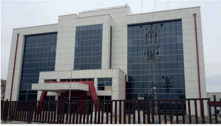
Suşehri State Hospital with 50 Beds / SİVAS 9 Elevators, Rated Load: 1000 / 1600 kg
