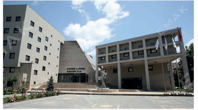
Kayseri and Its Vicinity Electricity T.A.Ş. / KAYSERİ Rated Load: 800 kg
