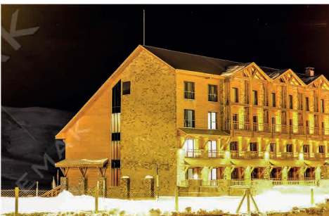
Magna Pivot Hotel / KAYSERİ 2 Elevators, Rated Load: 800 kg
