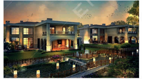
Meliketna Villas / KAYSERİ 2 Elevators, Rated Load: 450 kg
