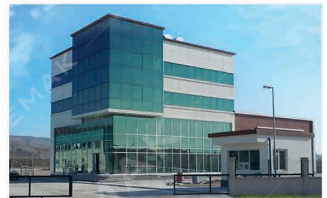
Mobitek / KAYSERİ 2 Elevators, Rated Load: 800 kg
