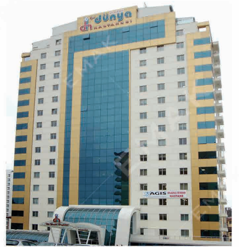
Dünyam Hospital / KAYSERİ 8 Elevators, Rated Load: 2000 kg
