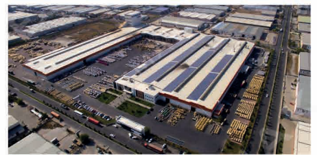
Haşcelik / KAYSERİ 3 Elevators, Rated Load: 800 / 3000 kg
