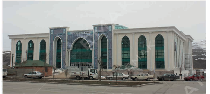
Semerkand Cultural Center / ANKARA 9 Elevators, Rated Load: 400 / 630 kg
