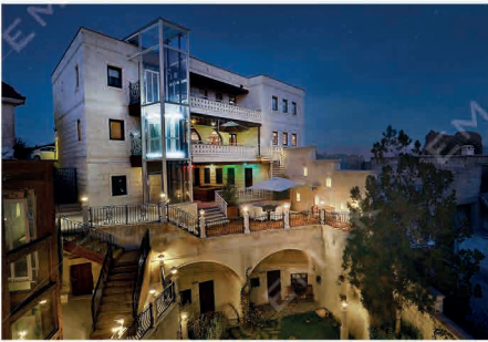
Satrapia Hotel / NEVŞEHİR 2 Elevators, Rated Load: 450 / 630 kg
