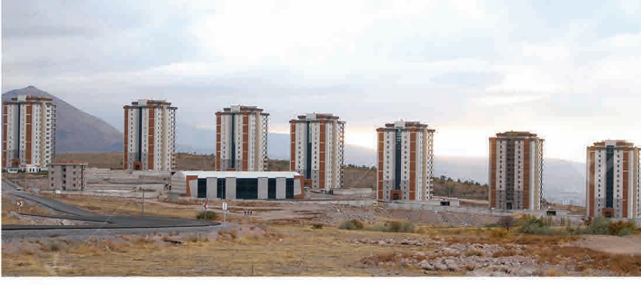
GulKent Complex / KAYSERİ 15 Elevators, Rated Load: 630 / 800 kg
