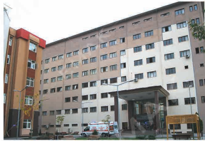
Erciyes University Heart Hospital / KAYSERİ 3 Elevators, Rated Load: 1600 kg
