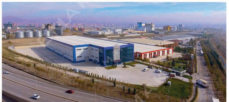
Seğmen Jam / ANKARA 5 Elevators, Rated Load: 450 / 3000 kg
