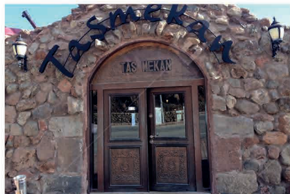
Taş Mekan Meat restaurant / KAYSERİ 2 Elevators, Rated Load: 800 kg
