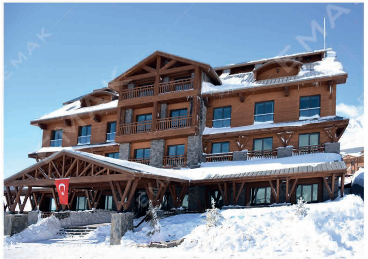
Magna Hotel / KAYSERİ 2 Elevators, Rated Load: 800 kg
