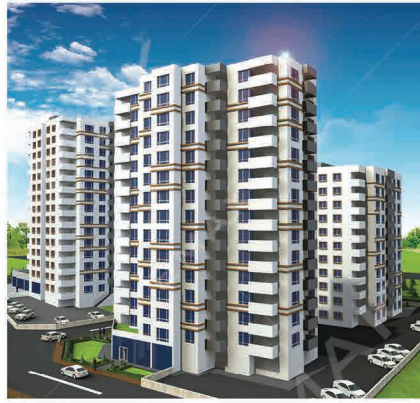
Ersu Construction Erkiilet / KAYSERİ 8 Elevators, Rated Load: 800 kg
