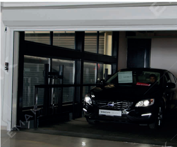
Volvo Showroom EMAK Cargo Platform Rated Load: 2 Tons
