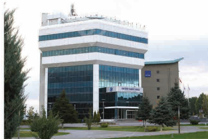
Kayseri Chamber of Industry / KAYSERİ 2 Elevators, Rated Load: 630 kg
