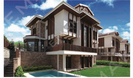
Villas in Cappadocia / ANKARA 32 Elevators, Rated Load: 400 kg
