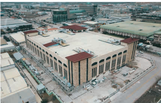
Baklavacı Hacibaba Factory / ANKARA 4 Elevators, Rated Load: 800 / 3000 kg
