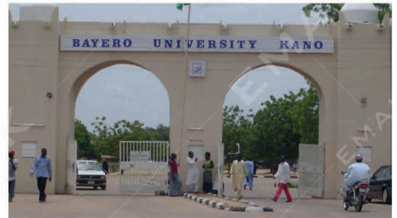
Bayero University Kano – Kano / NIGERIA 7 Elevators Panoramic Rated Load: 1000 Kg
