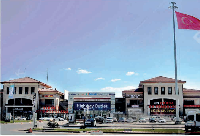
HighWay AVM / BOLU 13 Elevators, Rated Load: 1000 kg
