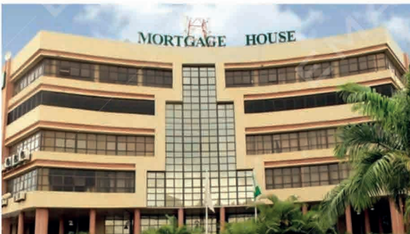
Federal Mortgage Bank – Abuja / NIGERIA Panoramic, Rated Load: 1000 Kg
