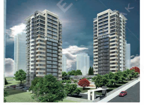
EvrenPark / Ankara 4 Elevators, Rated Load: 800 kg
