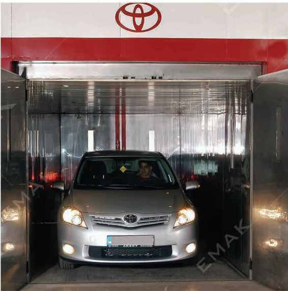
Toyota Showroom EMAK Cargo Elevator Rated Load: 2 Tons
