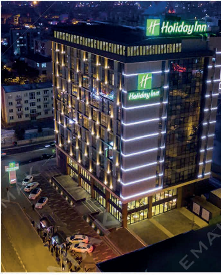
Holiday Inn Hotel / KAYSERİ 2 Elevators, Rated Load: 250 / 4000 kg
