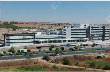
State Hospital with 300 Beds / GAZİANTEP 13 Elevators, Rated Load: 630 / 1600 kg
