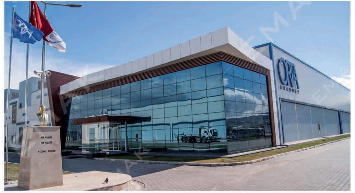
Orta Anadolu Factory / KAYSERİ 2 Elevators, Rated Load: 1300 kg
