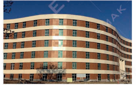
Etimesgut State Hospital with 250 Beds / ANKARA 11 Elevators, Rated Load: 450 / 1600 kg
