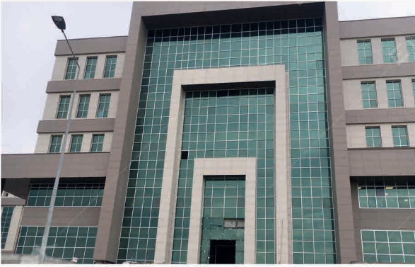
Courthouse / TEKİRDAĞ 15 Elevators, Rated Load: 800 kg
