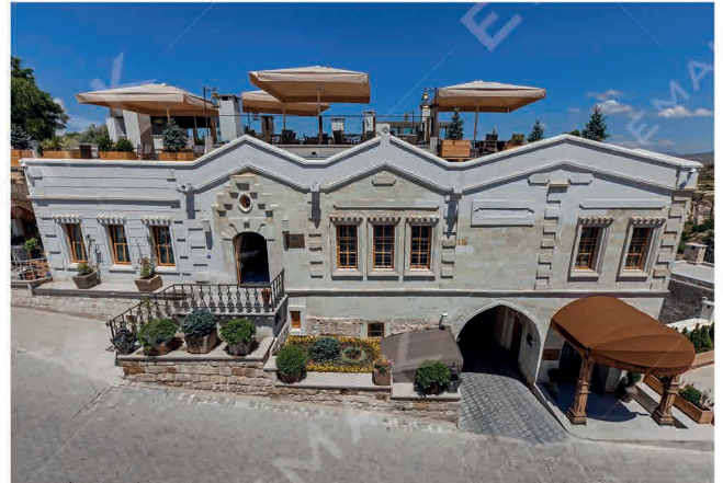
The House Hotel / NEVŞEHİR 2 Elevators, Rated Load: 250 / 630 kg
